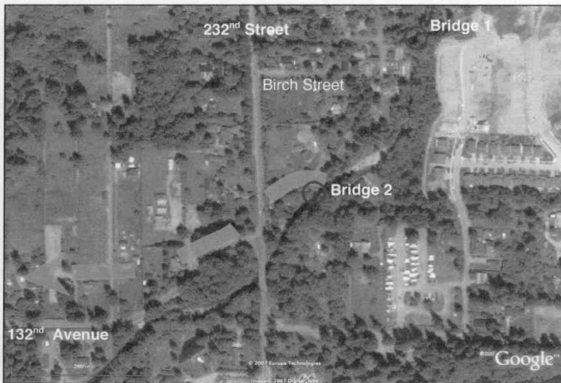
Figure 4: Aerial image of the area where flooding initiated, showing various features and the approximate path of flood waters- they continued for several hundred more metres to the west.
